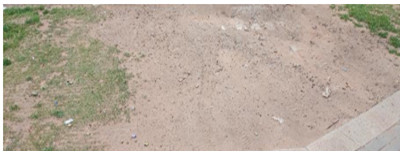
Example illegal driveway crossing
